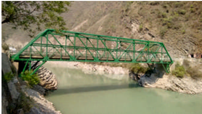
Retrofitting and strengthening of Zero bridge 64 m / 48 m at Tehri, 2002
