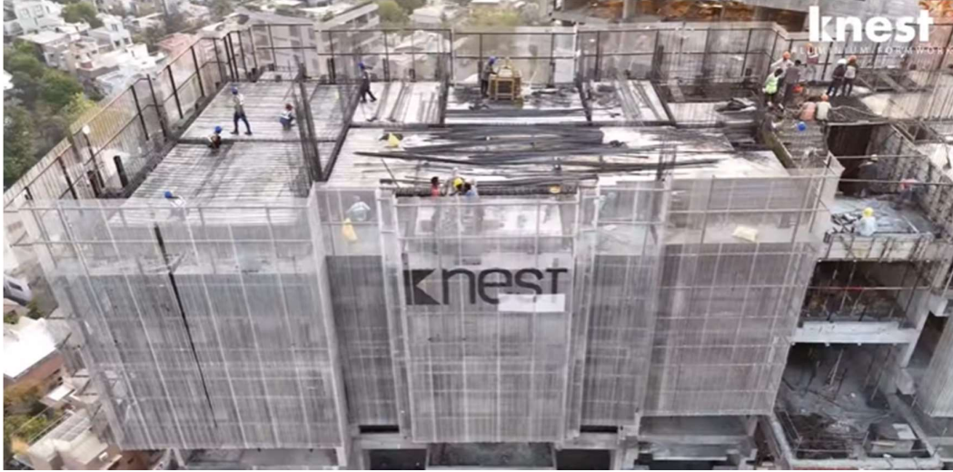
Fig 3: Setup of Working Platform with PSS (on site image).
