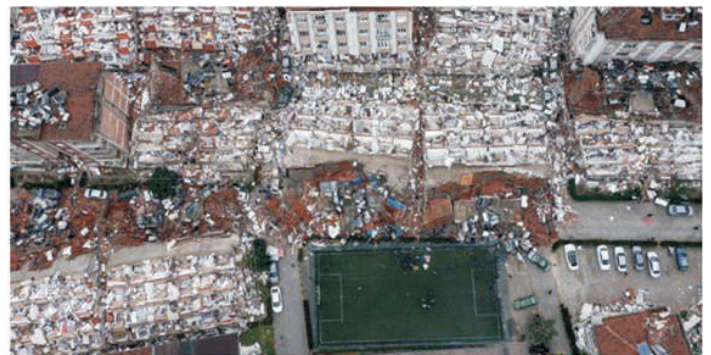
Figure 16. Pancake collapsed buildings in Hatay. Credit: IMO, 2023
