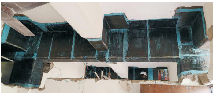
Fig 1.5.4: Beam Strengthening with CFRP wrapping
