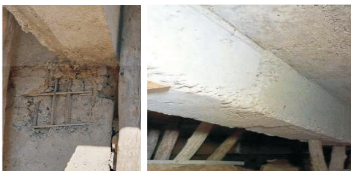
Fig 1.3.2: Rebar exposure and honeycombing in concrete
