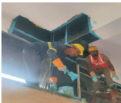
Fig 1.5.5: Column-Beam junction confinement with CFRP
