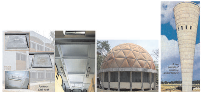
Several examples of shell and spatial structures at SERC, developed under the guidance of Prof. GSR (a) Funicular shell roof for the Concrete Testing Laboratory (CTL) building, (b) A 12.2m-diameter modified Füller dome made of light aluminium alloy tubes, and a 21 m tall mushroom-shaped water tank of 140000-litre capacity, designed as a hyperboloid of revolution
