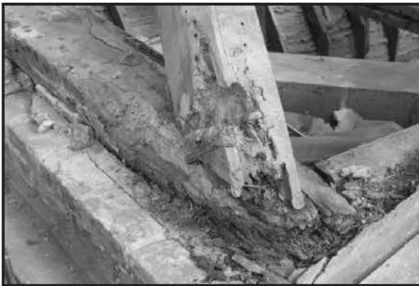
fig. 8. Fungus Attack Causing Brown Rot Of The Roof Rafter
