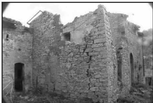
Fig. 18. Earthquake Affected Stone Masonry Structure
