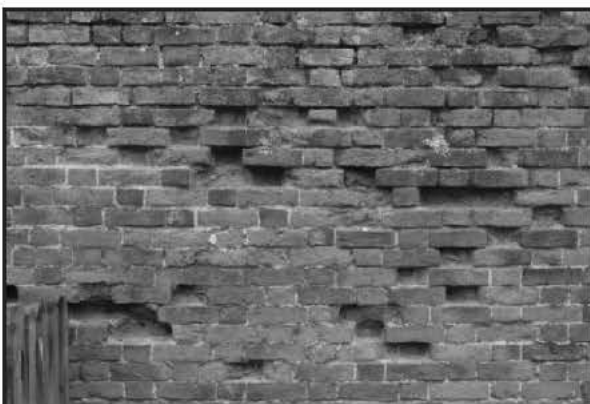
Fig. 9. Ivy And Masonry Bee Damage The Historic Brickwork
