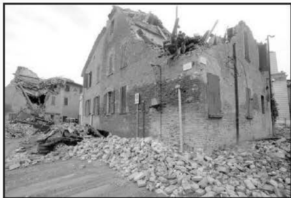
Fig. 17. Earthquake Affected Brick Masonry Structure
