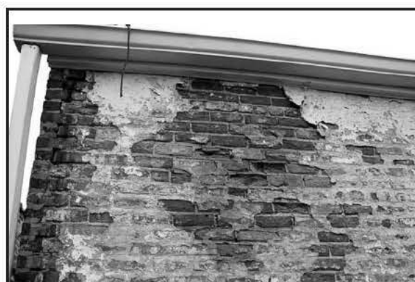
Fig. 14. Deterioration Of Brick Masonry
