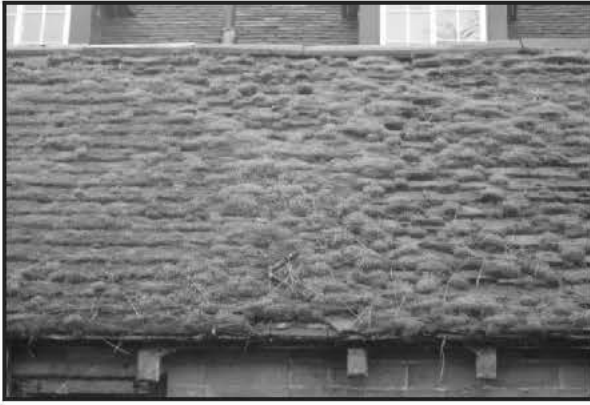
Fig. 7. Moss Damages Roof Due To Its Weight, Water Retention & Lifting Of Tiles
