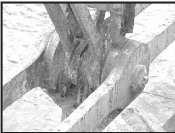
Fig. 4. Corrosion Of Structural Steel
