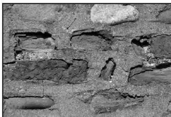
Fig. 16. Spalling Of Stone In A Historic Wall Due To The Inappropriate Use Of Hard Cement Mortar
