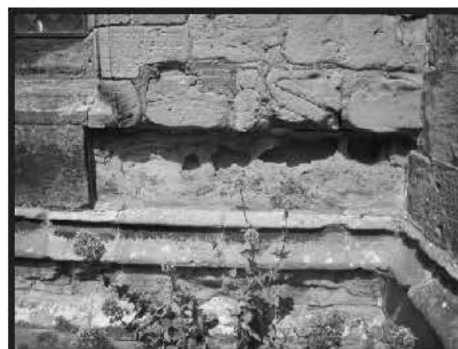
Fig. 2. Damaged Stonework Caused By Combination Of Factors - Dust Particle Erosion, Soft Or Poor Quality Stone, Heat & Wind
