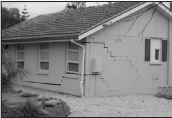
Fig. 3. Failure Of Structure Due To Settlement In Foundation
