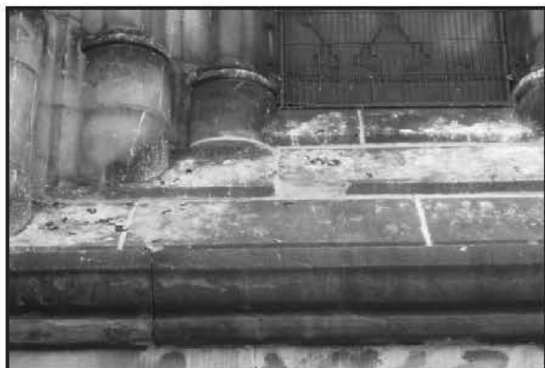
Fig. 13. Bird Droppings - Heavily Soiled Stonework
