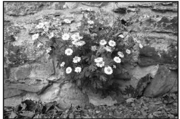
Fig. 6. Daisies Growing In An Area Of Damaged Mortar On A Historic Wall
