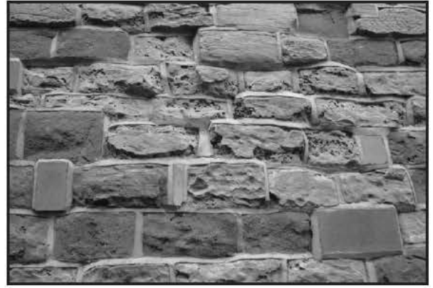
Fig. 10. Damage To A Historic Wall Caused By Masonry Bees, An Inappropriate Pointing Style And Hard Cement Mortar
