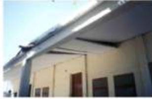
Figure 14-10. Type B damage — roof planks slipped.
