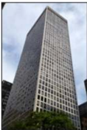
Fig. 1 The revolutionary framed-tube structural system of Chestnut De-Witt apartment building, at Chicago (Photo: Anuthama Srisailam)
