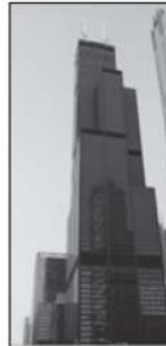
Fig. 4 Willis Tower, Chicago introduced the bundled tube structural system (Photo: Karthik Muthusamy)
