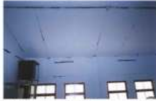
Figure 14-12. Type D damage — minor opening of grouted joints.
