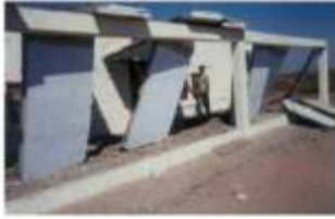
Figure 14-9. Type A damage — major damage to structure.
