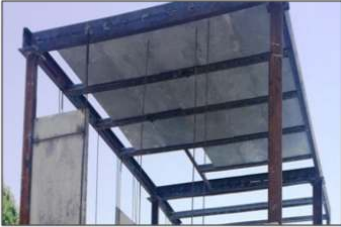
Fig.No.6: Slab Panel Over Bridge.
