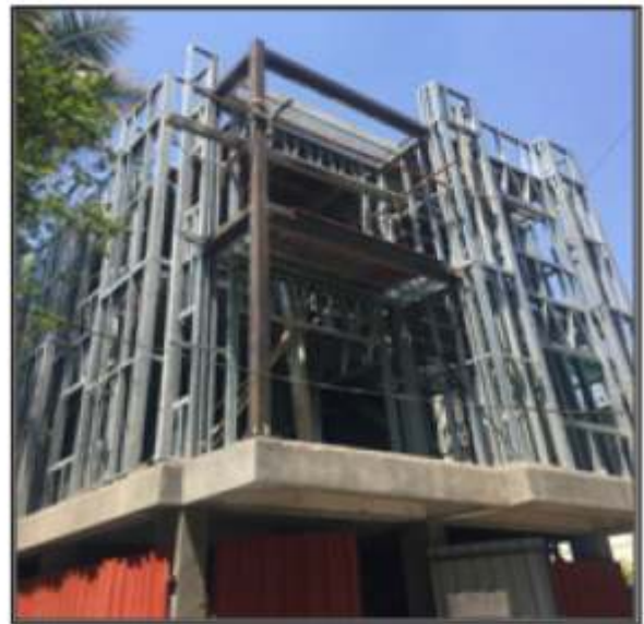
Fig. No. 1: Light Gauge Steel Frame (G+2) 15,000Sq.ft. Internal & External Walling.
