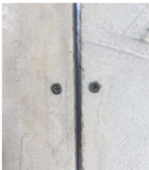
Fig.No. 8 : Fixing of panels with Self tapping screw
