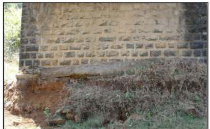
Erosion of soil below the abutment
