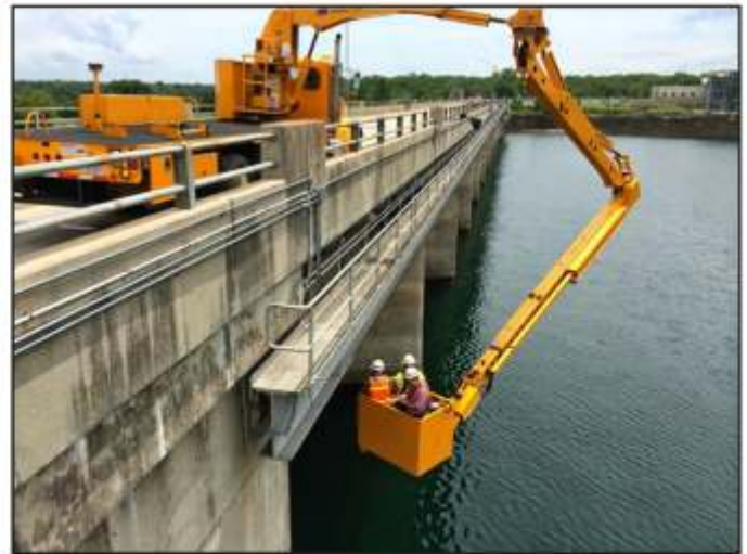
Inspection of inaccessible portion of bridges
