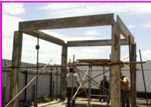
Fig. No. 6 : Erection Sequence Col. Beam & Slab
