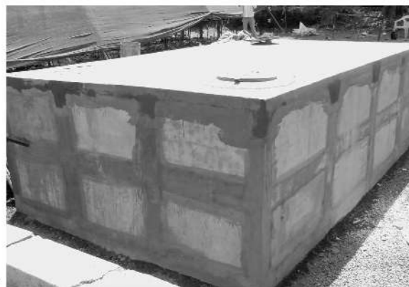
Tank Size. 6 x 3.6 x 1.8 mtrs ht., 40000 ltr capacity
