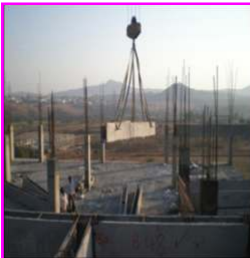
Fig.No. 3 : Lifting of Beam
