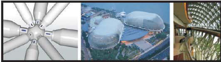
Fig. 26 MERO system: (a) KK-Ball node system, (b) and (c) Singapore Arts Center built in 2002 (source: http://en.wikipedia.org/ )
