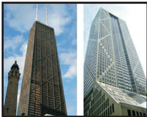
Fig. 33 Elegant skyscrapers designed by Khan using innovative structural systems (a) John Hancock Center, (b) the Onterie Center (photo: Author)
