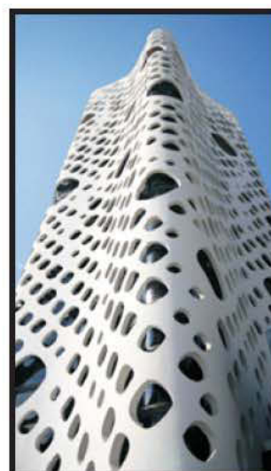
Fig. 35 Buildings with diagrid system: (a) the Gherkin at London (b) Hearst Headquarters at New York (c) The O-14 Building in Dubai [Source: (a) & (b) http://en.wikipedia.org/ , (c) Reiser et al (2010)]
