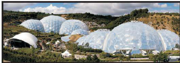
Fig. 27 Double layer intersecting domes of Eden project at Cornwall, U.K., built in 2000 (source: http://en.wikipedia.org/ )
