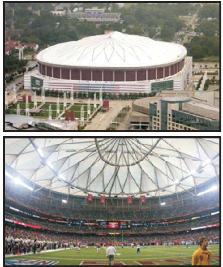
Fig. 31 The 256 m diameter Georgia Dome in Atlanta designed by Matthys Levy, 1992 (a) External view, (b) Internal view (source: http://www.stadiumsofprofootball.com/ )
