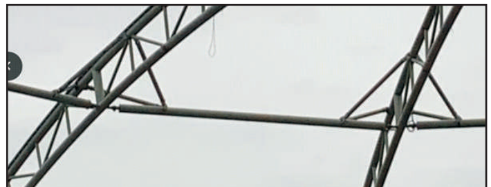
Pinned connections between arch and intermediate ring
