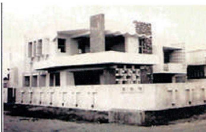
An overhead water tank designed by a new method developed by Dr Ramakrishnan, resulted in cost savings of 30% and Dr Ramakrishnan's first house in Coimbatore was a all-concrete building
