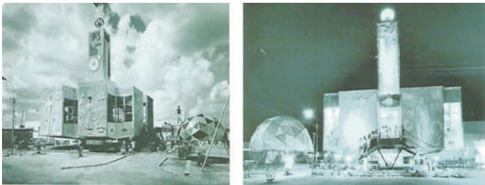
The PSG Pavilion at the International Industrial Exhibition, Madras built in 1968. This structure rises from water in the fountain to a height of 120 feet, symbolizing the Lotus flower, sacred in the Hindu mythology.
