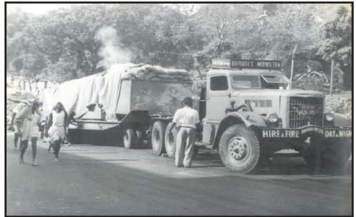
Kemps Corner Load Testing (1965)
