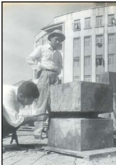
Inspection of concrete hinging Bombay Municipal Corporation
