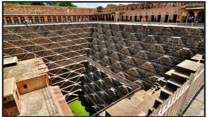
Fig-2a- On three sides steps are provided that lead down to the bottom of well.
