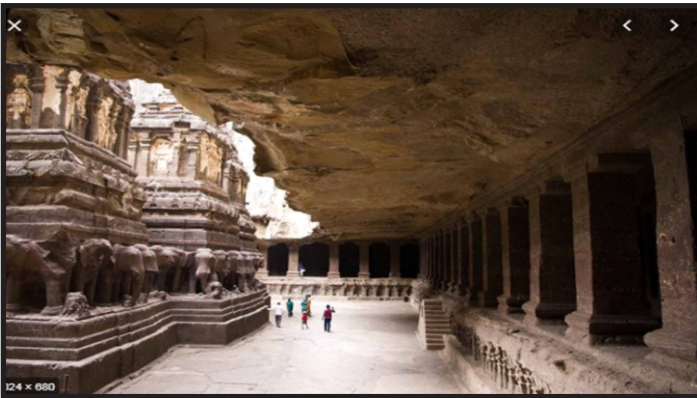
Fig-3b-A rare Rock mass 'Cantilever Canopy'-about 6m wide and 24m in Height is standing for past more than 1100 years.
