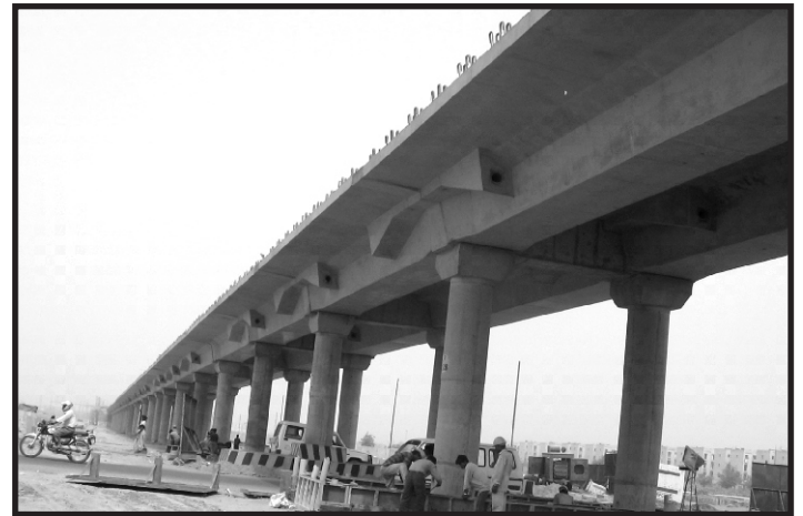
Fig. 4 (b) A view of II stage Stressing Blisters
