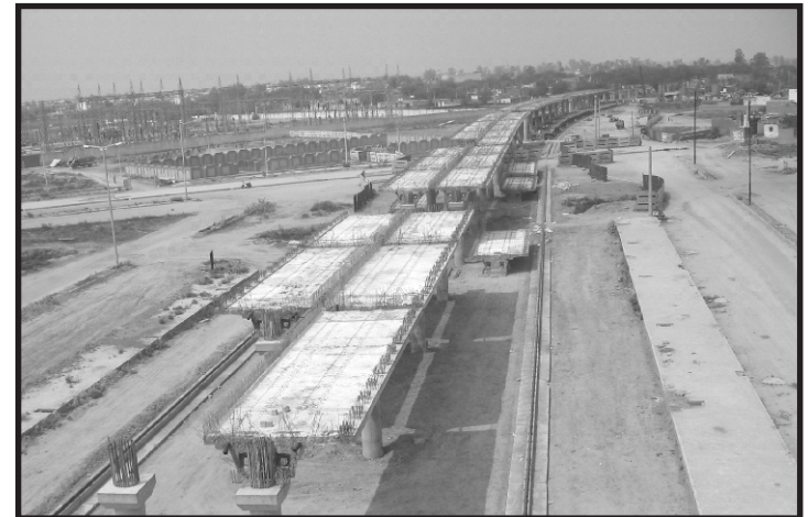
Fig. 5 (b) Box Girders Launched along the Curve Section
