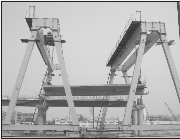
Fig. 5 (a) Precast Girder being Lowered
