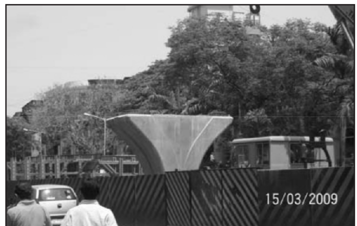
Concrete surface as seen above shall be surface of Inbuilt Ferro-cement Structural Formwork.
