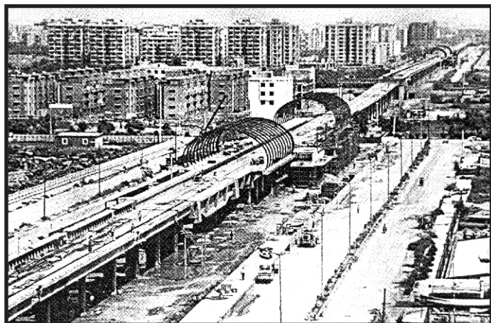
Fig. 8 Elevated Viaduct under construction
