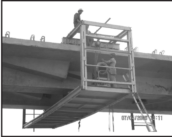
Fig. 4 (a) Platform in Position for II stage Blister Stressing
