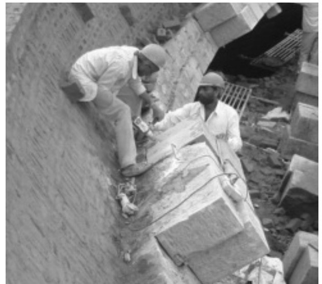
Photo 1: Fixing dome stone
