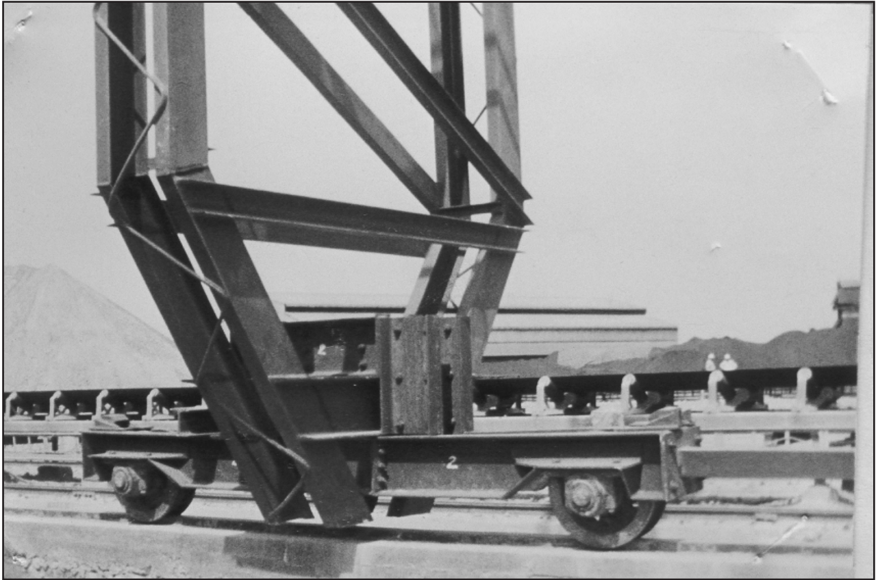
4 - Rolling the portals on wheels to required location
