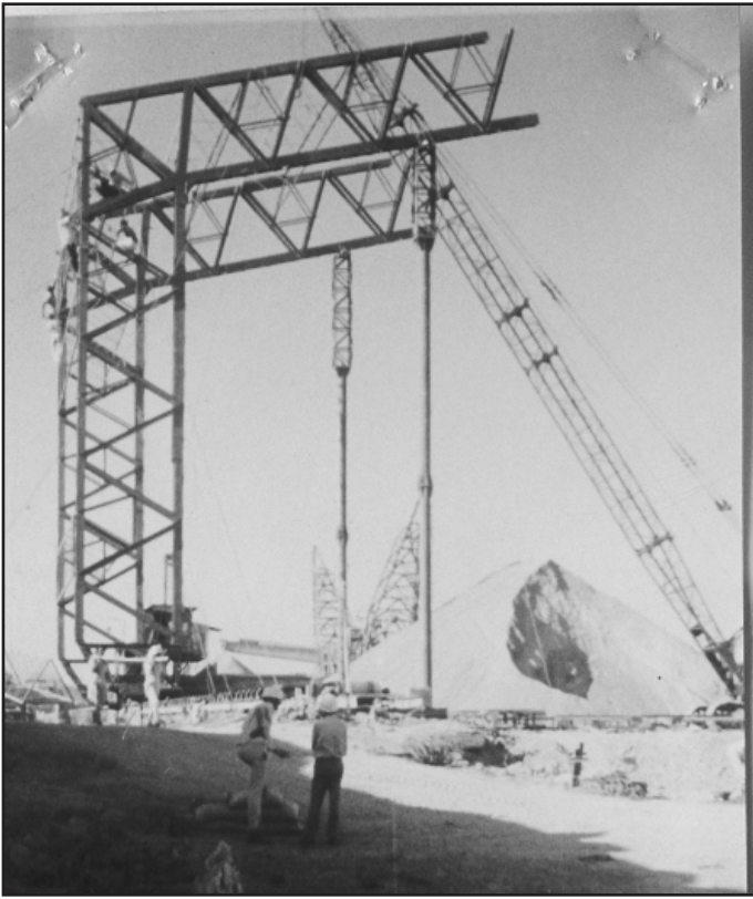
1 - Erection of frame with temporary support left side
