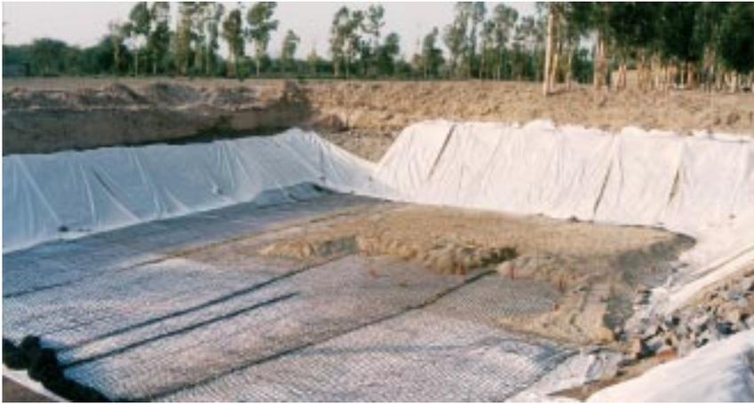
After scientific soil testing, the foundation of Swaminarayan Akshardham was made in accordance with an ancient Indian technique. Layers of sand, stone and geotextiles were laid to create a strong foundation.
