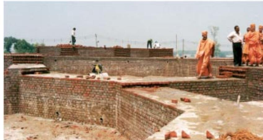
An iron-free foundation with a 42 feet high plinth of 5 million bricks was built. The internal connections of the hexagonal shaped brick plinth added to its strength
