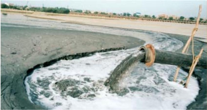
The land was with large 10 ft deep craters. To fill up the craters and level the land would have required one year to accomplish. But it was accomplished in only six months by channeling the excess silt of river Yamuna.
