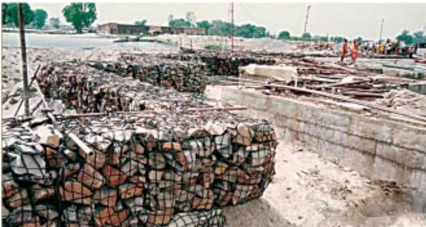
With the possibility of earthquakes care was taken to build a robust foundation, by considering soil porosity and the seismic forces.
