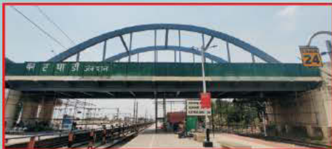
STRENGTHENING OF KATPADI BRIDGE AT TAMIL NADU
