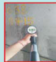
CAPO TEST FOR CONCRETE STRUCTURE
