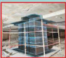
COLUMN STRENGTHENING USING CFRP AT PUNE
