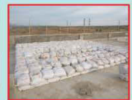
SLAB LOAD TESTING USING SANDBAGS
