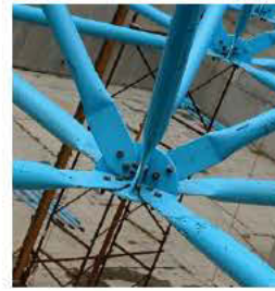
Snap shot of plate connector used in space frame
