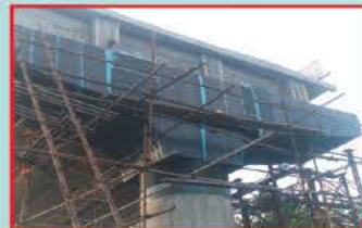
PIER STRENGTHENING AT KERELA
