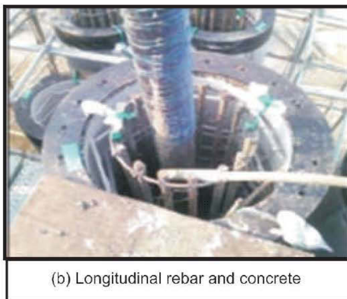
Fig. 1 Reinforcement of large diameter PHC pile
