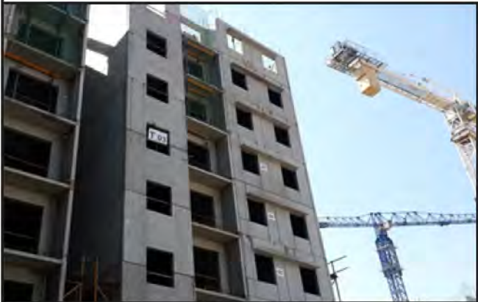
Precast construction at Peenya, Bangalore – Tata housing under erection
