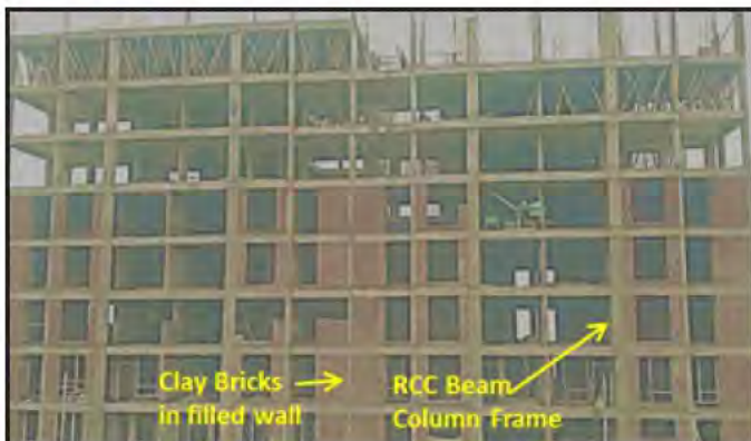
Conventional construction technology – beam column frame with red brick infill wall
