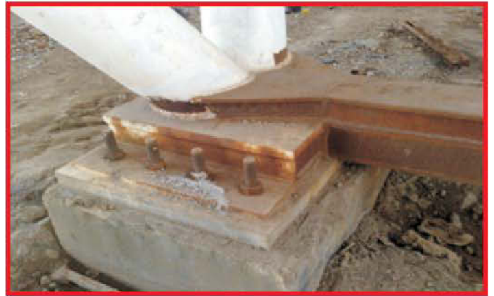
Fig.15: Column Base & Strut
