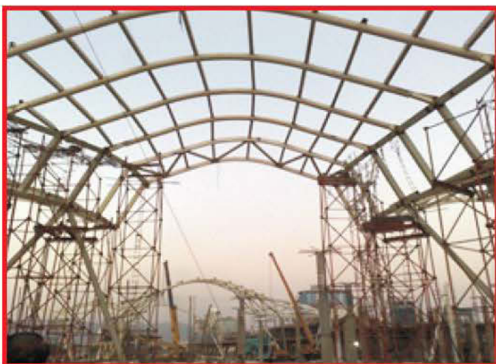
Fig.14: Under Construction with temporary support's & staging
