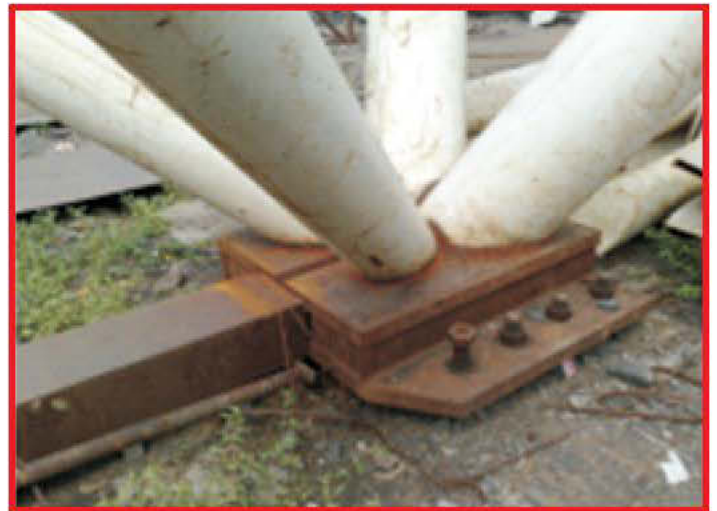
Fig.13: CHS Profile Cutting
