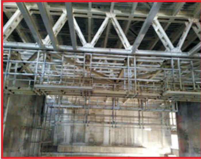
Fig 37 – Suspended platforms from the underside of Auditorium trusses
