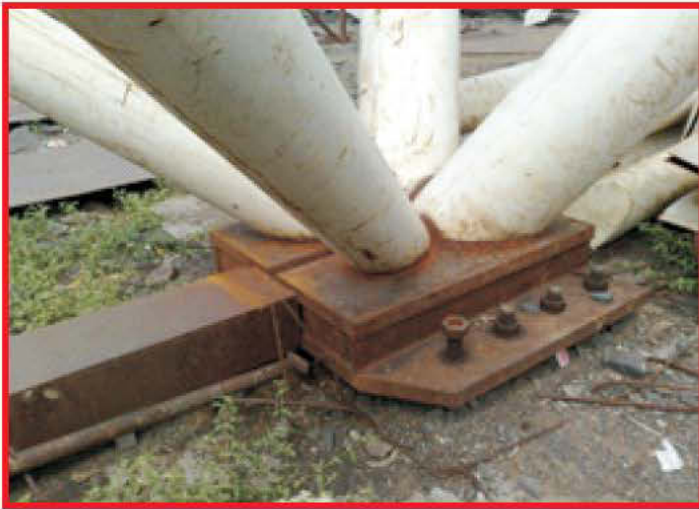
Fig.15: Column Base & Strut
