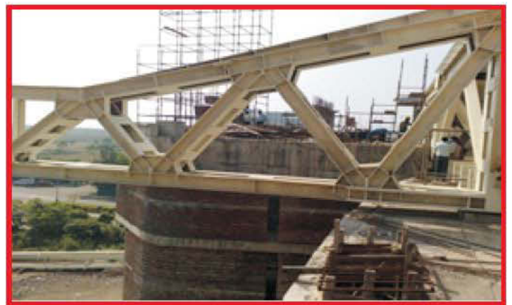
Fig.34: Auditorium Roof Truss under construction
