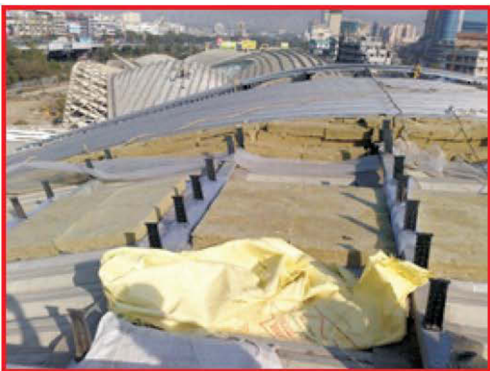
Fig. 22: Views from Top of Roof showing the double skin in foreground - Steel Decking below, Insulation, clips (black color) and aluminium top skin laid in one piece end-to - end on curve
