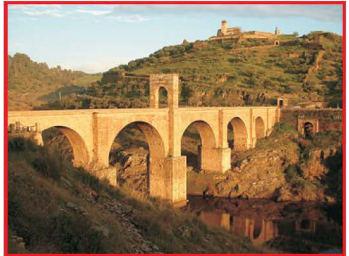
Fig.1 Alcántara Bridge at Alcántara, Spain built between 104 and 106 AD by an order of the Roman Emperor Trajan
