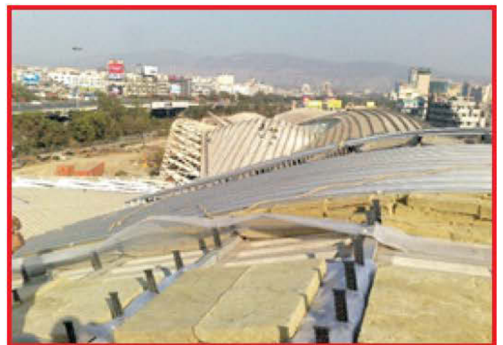
Fig. 22: Views from Top of Roof showing the double skin in foreground - Steel Decking below, Insulation, clips (black color) and aluminium top skin laid in one piece end-to - end on curve
