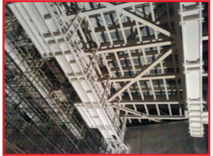
Fig 37 – Suspended platforms from the underside of Auditorium trusses
