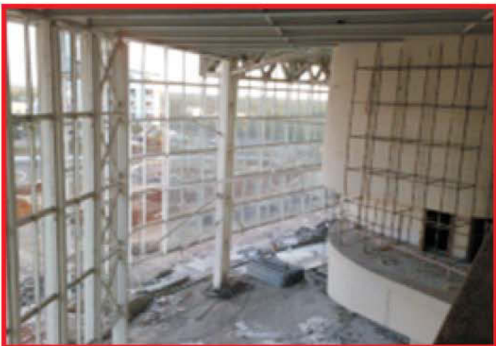
Fig. 36: Views of Foyer Suspended Glazing and bracings
