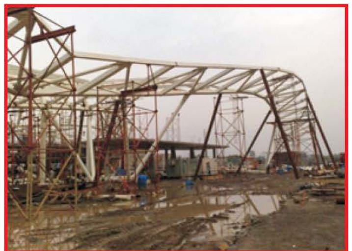
Fig.14: Under Construction with temporary support's & staging
