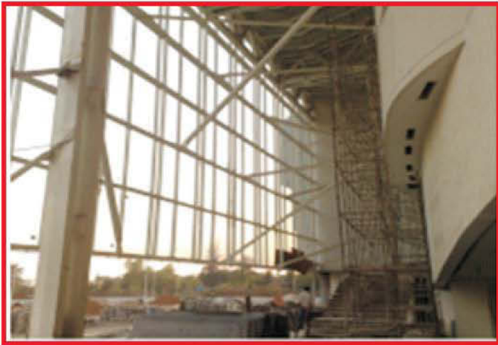
Fig.35: Lenticular Truss after erection
