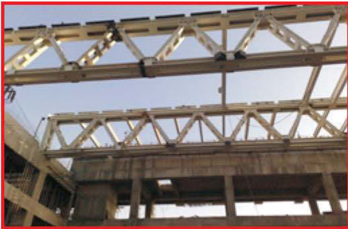
Fig.34: Auditorium Roof Truss under construction
