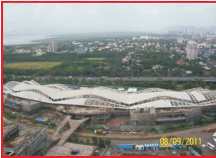
Fig.19: Under Construction with steel decking on Roof partly erected
