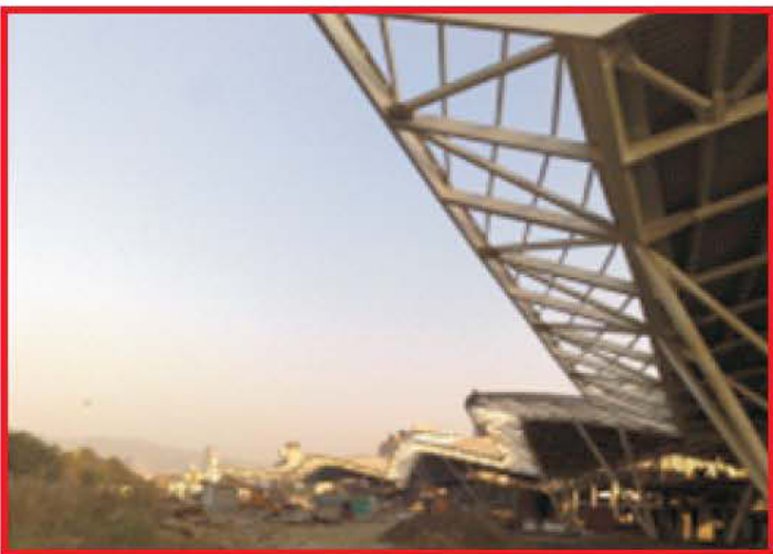
Fig.19: Under Construction with steel decking on Roof partly erected
