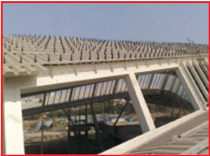
Fig. 21: Views from Top of Steel Decking - lower skin
