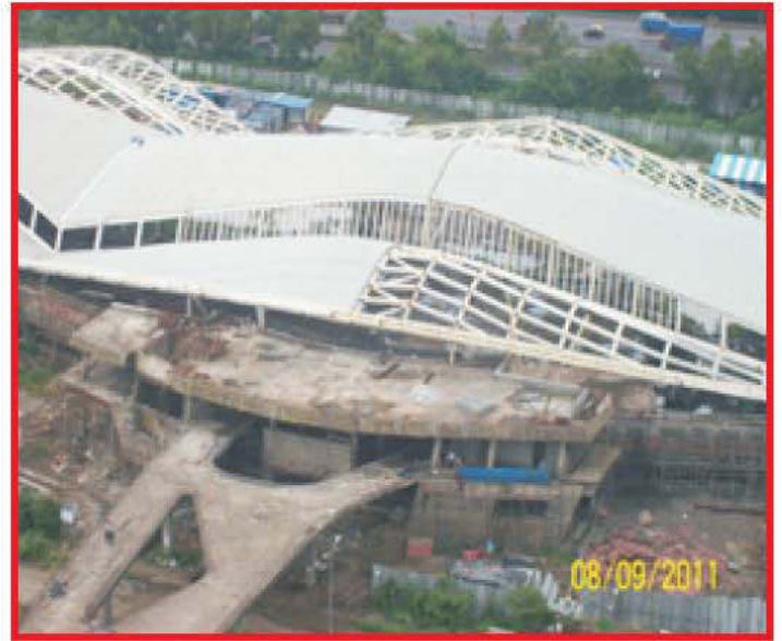
Fig.19: Under Construction with steel decking on Roof partly erected
