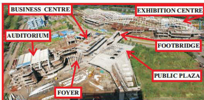
Fig.1b: Over all view – Under construction
