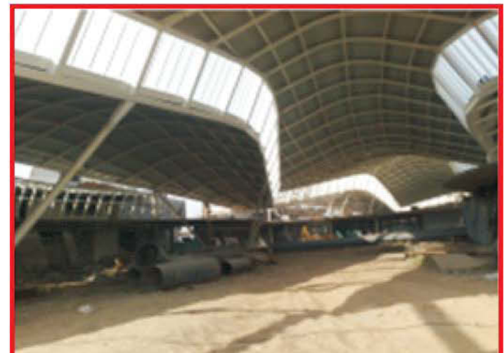
Fig.19: Under Construction with steel decking on Roof partly erected
