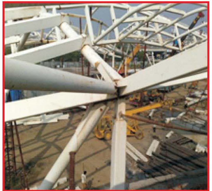
Fig.16: Column Truss Connection
