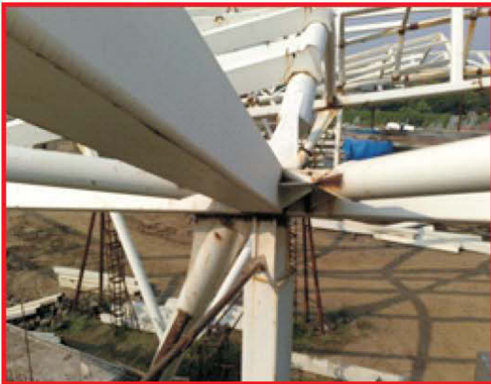
Fig.16: Column Truss Connection
