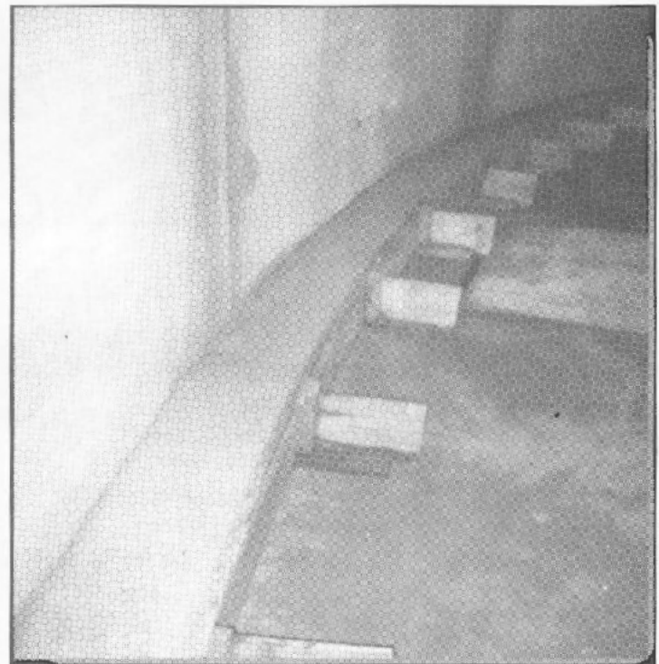
Figure 9: Waterstop Embedded in Footing
