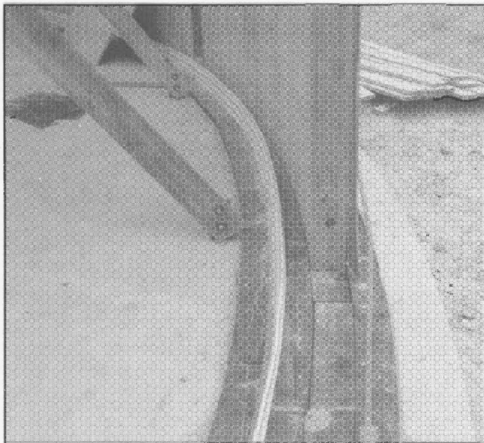
Figure 14a: Wall Panel Set on Bearing Pads
