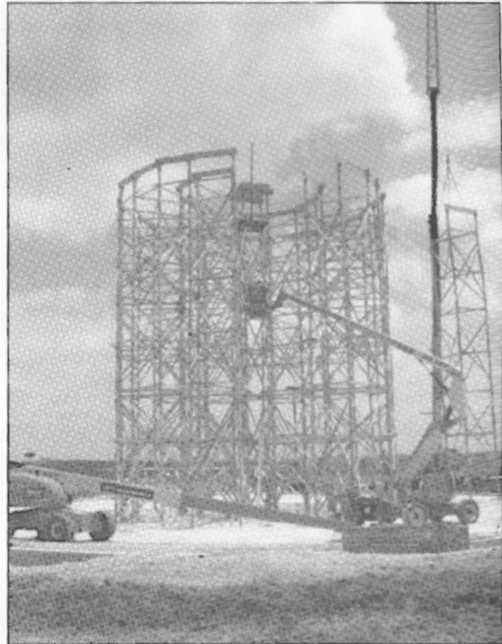
Figure 20: Falsework for Dome Construction
