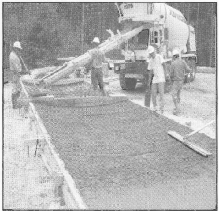
Figure 12: Panel Casting and Finishing
