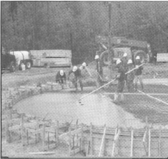
Figure 7: Screeding and Finishing Operation
