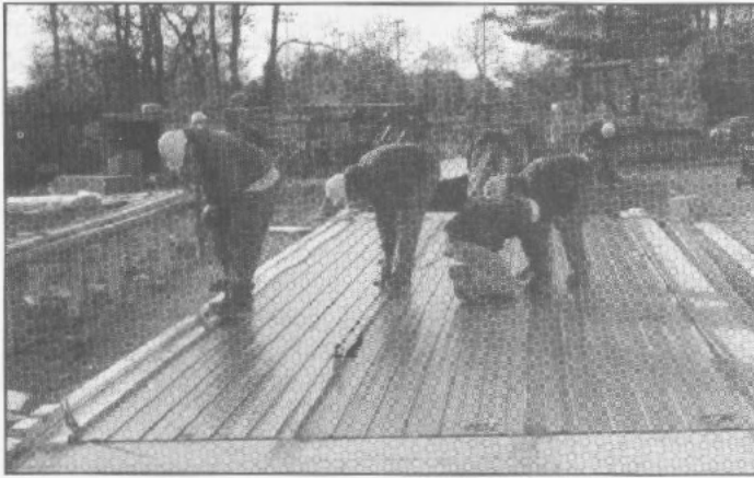
Figure 11: Diaphragm for Wall Panels
