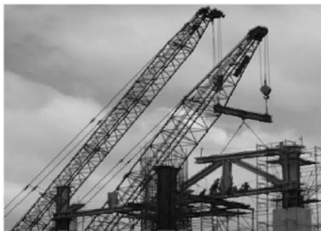
TRANSFER GIRDERS DURING ERECTION
