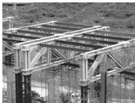
TRANSFER GIRDERS AFTER ERECTION
