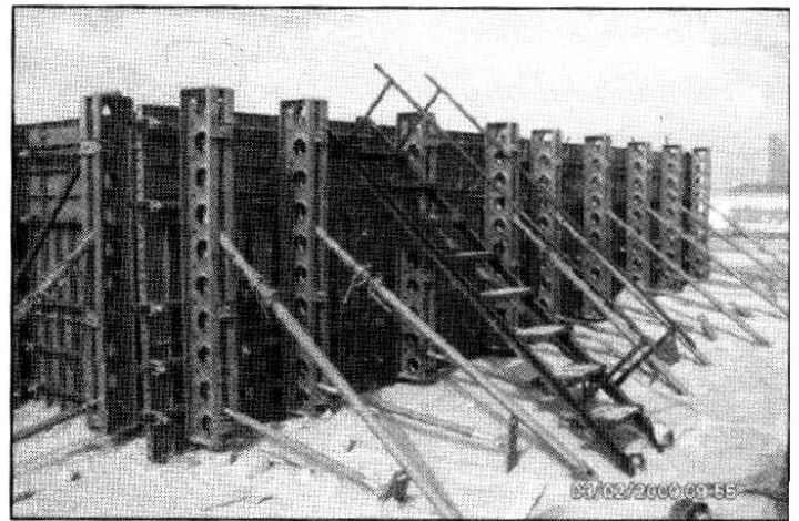
Fig-3b – Pile-cap formwork (M/s RMD Kwikform type)
