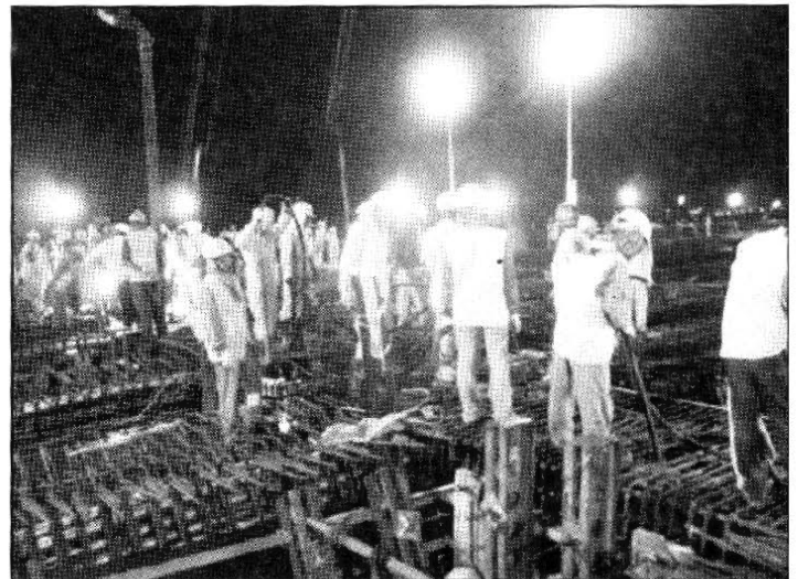
Fig-12. Due to heat in summer, night concreting of the Large deck was preferable
