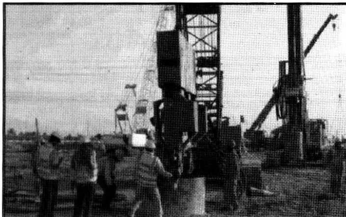
Fig-3a – Pile Driving in progress
