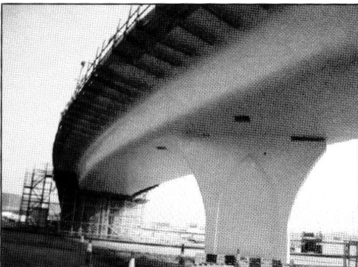
Fig-10. MDN-1A on verge of completion. The white epoxy coating can be easily seen.
